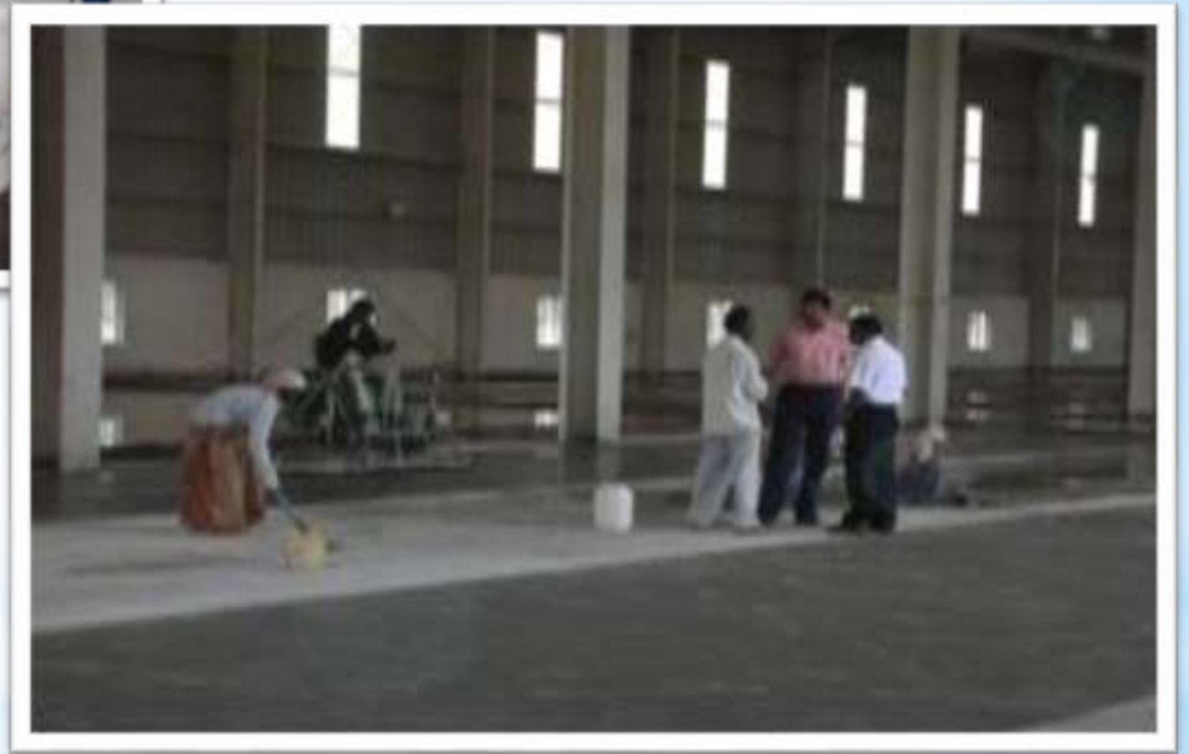
Monton Hydraulic Project Site At Cholavaram Chennai.
